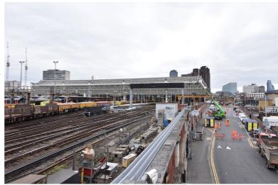
The new signalling gantry now extends over platforms 1-8, and has been carried out ahead of work to extend platforms 1-4, which Network Rail will undertake during a three-and-a-half week part-closure of Waterloo station in August 2017.
